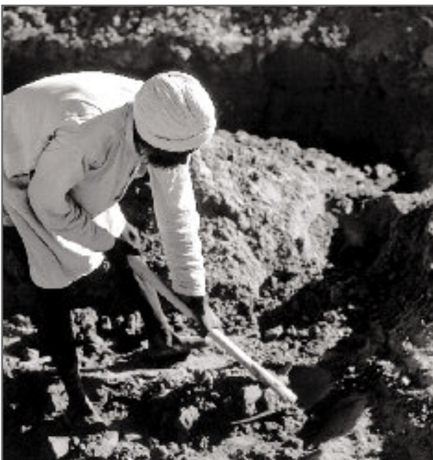
Digging clay to make bricks for walls and houses
